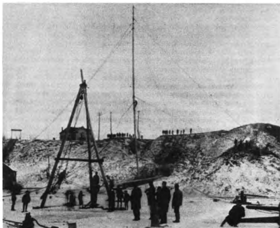
Another view showing the erection of the antenna masts for the DeForest Wireless Telegraph Co. of Canada wireless telegraph station at Hamilton Bay (Burlington Bay) Ontario in 1903, one of the first stations in Canada
